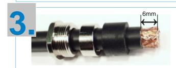
Remove 6 mm of the PVC sheath from the end of the cable with a knife.
