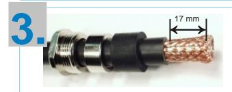
Remove 17 mm of the PVC sheath from the end of the cable with a knife.
